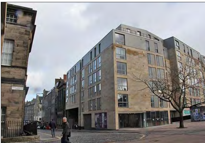
New student accommodation, South College Street
