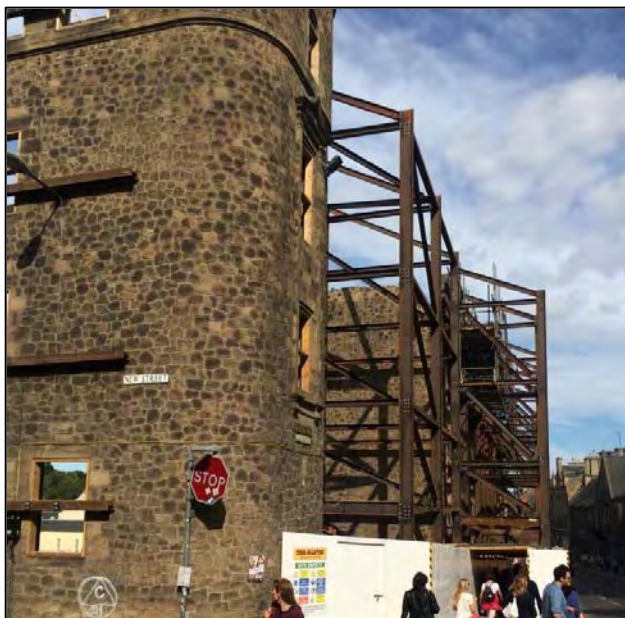
'New Waverley' development, the Canongate
